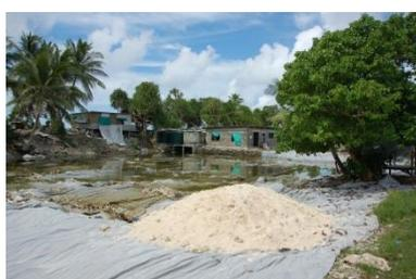
Pits drained and with the lining in place to stop the sand sinking once it is put into the hole
