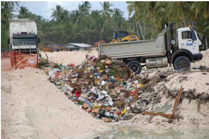
The Funafuti rubbish tip after it has been compacted and buried under dredged sand as part of the NZ Borrow Pits Project. This method for tidying up the tip will only work once...
